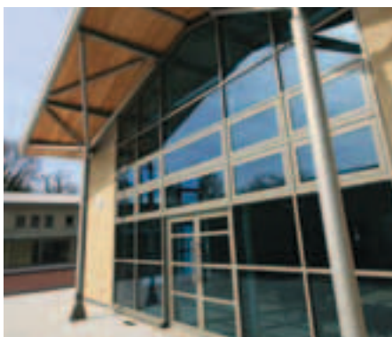
A new flagship training centre for the Territorial Army and Army Cadet Force at Cwrt-y-Gollen near Crickhowell. The prime users are B Squadron 203 (Welsh) Field Hospital and Gwent and Powys Army Cadet Force. The facility provides a modern training establishment as well as being ideally located for outdoor activities in the Black Mountains and the Brecon Beacons.
