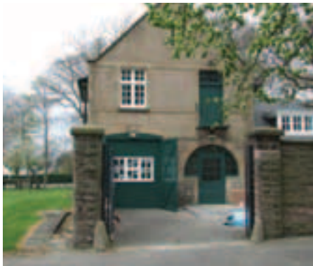
Existing building transferred from Regular Estate to Lowland RFCA, in sound structural condition and refurbished as new. Now the permanent HQ for training and administrative staff for Reserve Forces & Cadets Pipes & Drums completed 31st March 2009. Fully funded from RGI.
